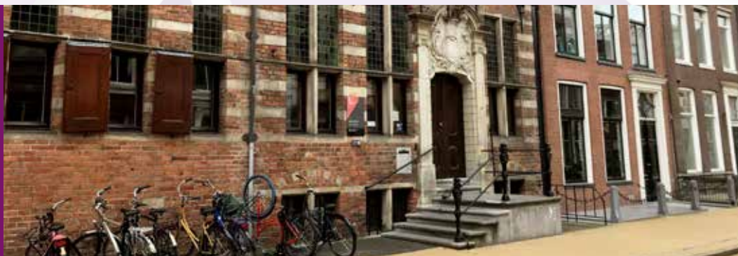
Building of the Faculty of Religion, Culture and Society. (RCS) Address: Oude Boteringestraat 38, 9712 GK Groningen.
